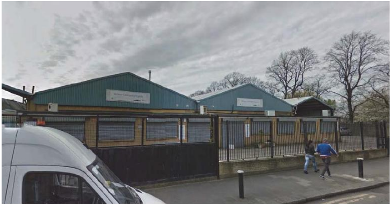
Photo of the existing building viewed from the front
